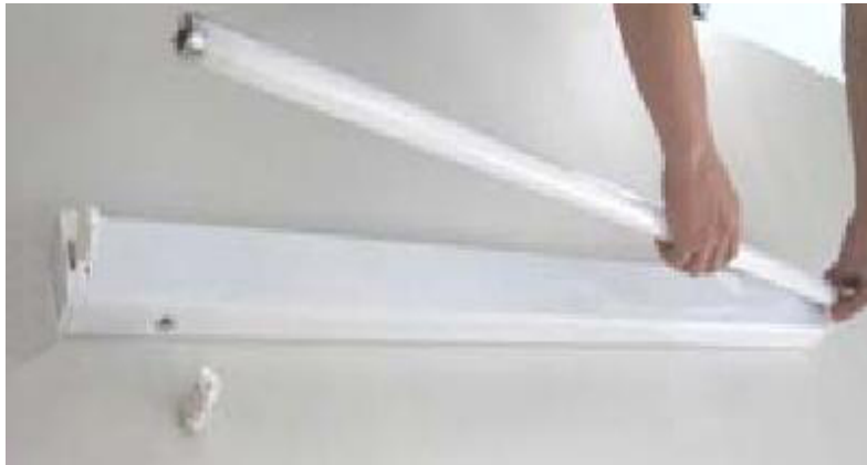
Remove the fluorescent tube (4)
